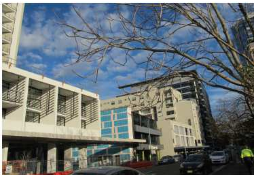
Figure 4 Street view subject site viewed from north east
